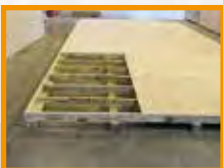
Pressure Treated Skids and Floor Joists
