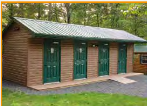
13x28 Campground Bathhouse
