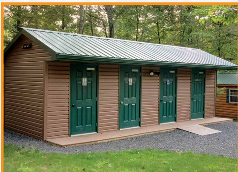
13x28 Campground Bathhouse
