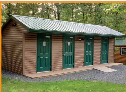
13x28 Campground Bathhouse
